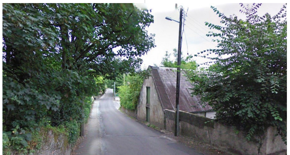
Figure 3: Mill building in 2011.
